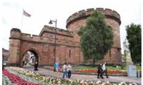
Above - Carlisle City Centre and Carlisle Citadel
