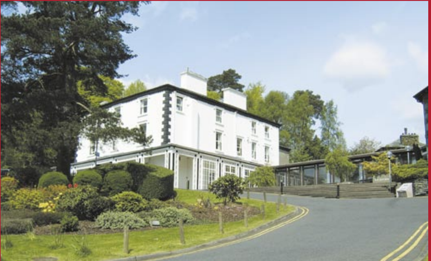
Scale How - the registry building at the Ambleside Campus
